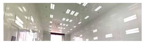
Modern technology has given way to improved lighting at reduced power. GFS engineers will help you develop a lighting layout in your booth that optimizes the lighting levels, as well as the number of fixtures and their location in the booth. To support the design process, GFS will also provide lighting calculations, which will show a graphic representation of the lighting levels you can expect in the booth.
