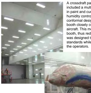
A crossdraft paint booth was ordered, and included a multi-mode control system to operate in paint and cure modes with temperature and humidity control. The booth was designed with conformal design, meaning the shape of the booth closely conforms to the shape of the aircraft. This method reduces total airflow in the booth, thus reducing energy use. The booth was designed to achieve high quality finish standards while protecting the environment and the operators.
