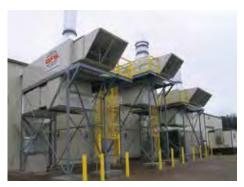
As air is exhausted from process equipment, heat is lost as well. Heat recovery systems are the answer to reclaiming some of the heat that escapes with the exhausted air, in turn providing measurable energy savings. On average, energy recovery systems provide 40-50% energy savings for air make-up systems serving the booth for both heating and cooling.
