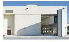
In some instances, such as new building construction, it is better to integrate the paint booth with the building elements. With a Hybrid Aircraft Paint Booth, the structure of the hanger holds up the booth ceiling and the building sidewalls can be integrated into the booth design to economize on material. GFS will work with the building architect(s) to integrate our paint booth design goals with the building design goals.
